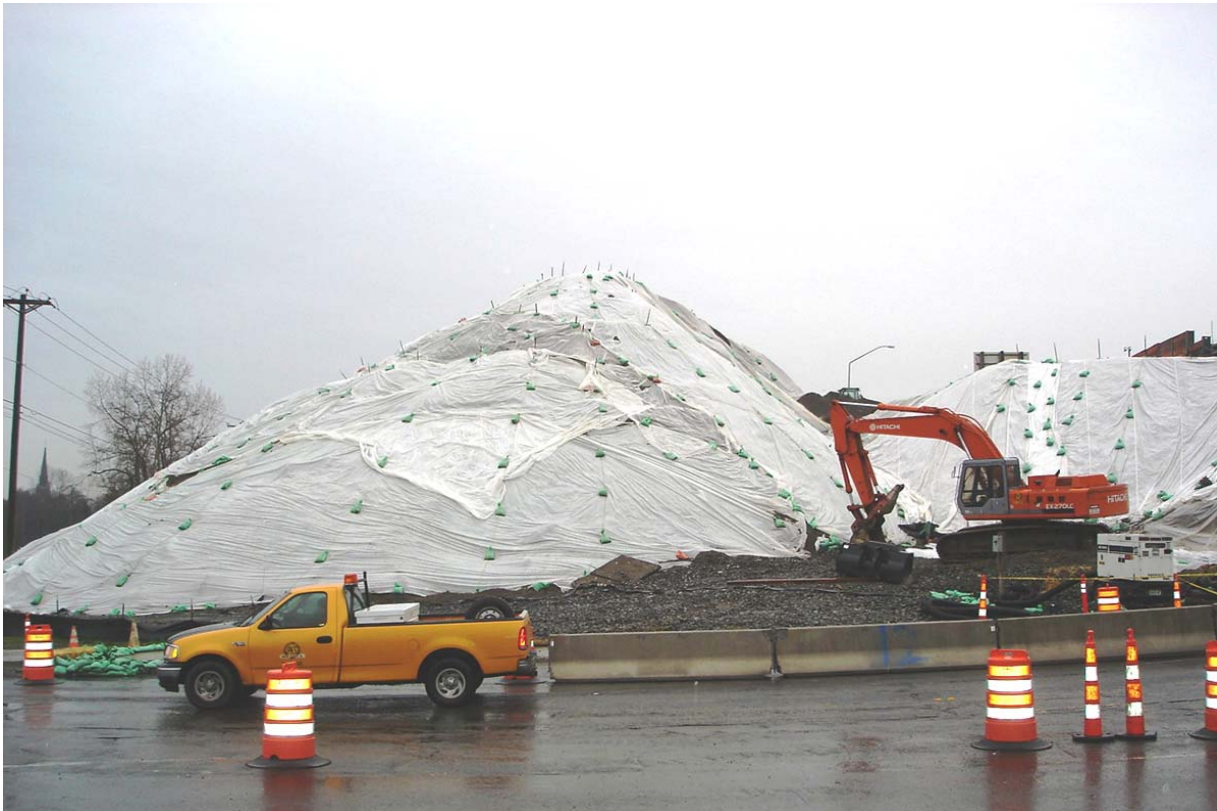
Figure 117. Material Covered with Plastic Sheetting
